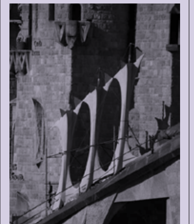
DEVELOPMENT OF THE COLONNADE DESIGN ABOVE THE NARTHEX (PASSION FAÇADE). THE COLUMNS HERE ARE PAINTED POLYSTYRENE PROTOTYPES MACHINED DIRECTLY FROM A 3D DIGITAL MODEL.
